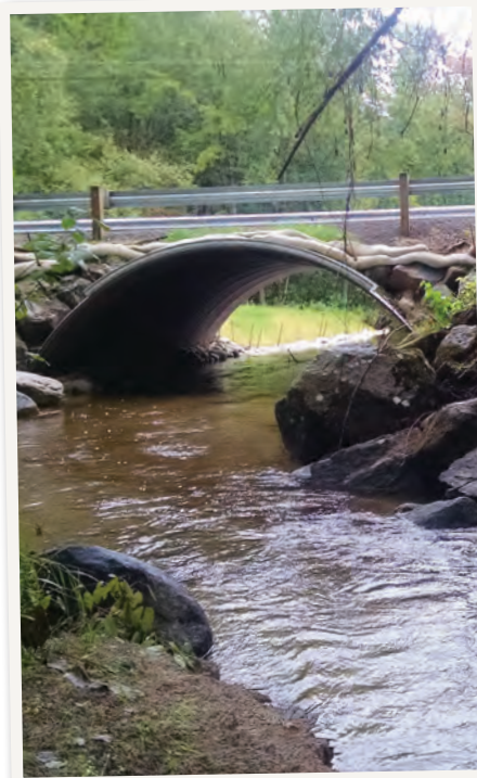
A wildlife-friendly arched culvert reconnects fish habitat on Falls Brook in Swanzey.
