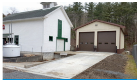
New feed and storage building at the Bath Hatchery
